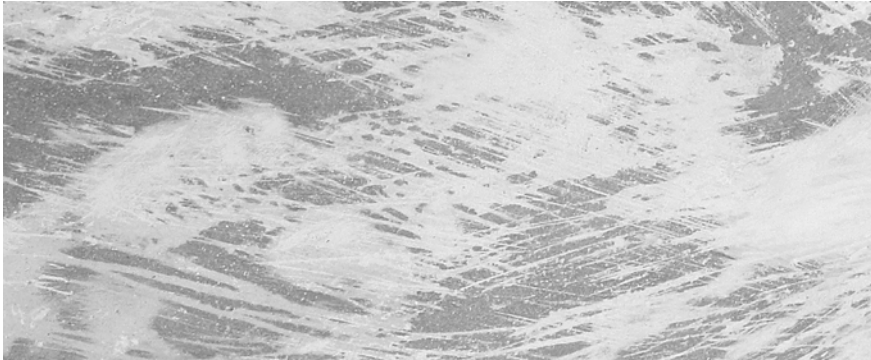
Detail of a concrete surface, where tool marks have been filled in with a lighter mix.
